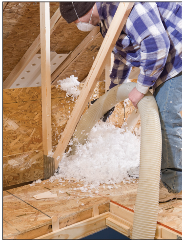
ADDING ATTIC INSULATION TO A RESIDENTIAL HOME
