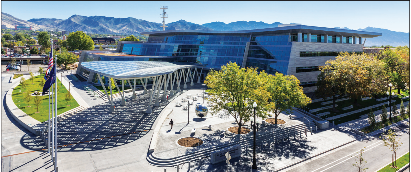
SALT LAKE CITY PUBLIC SAFETY BUILDING – NET ZERO DESIGN CREDIT: JEFF GOLDBERG
