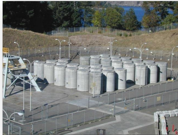
Independent spent fuel storage installation (left). Photo Credit: Portland General Electric Co. Spent fuel pool for storage of UNF (right). Photo Credit: San Onofre.
