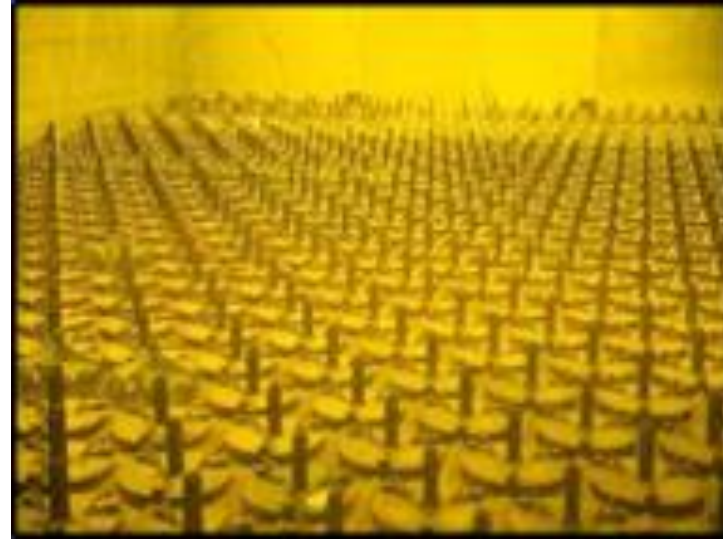
CPP-603 IFSF (Irradiated Fuel Storage Facility)
