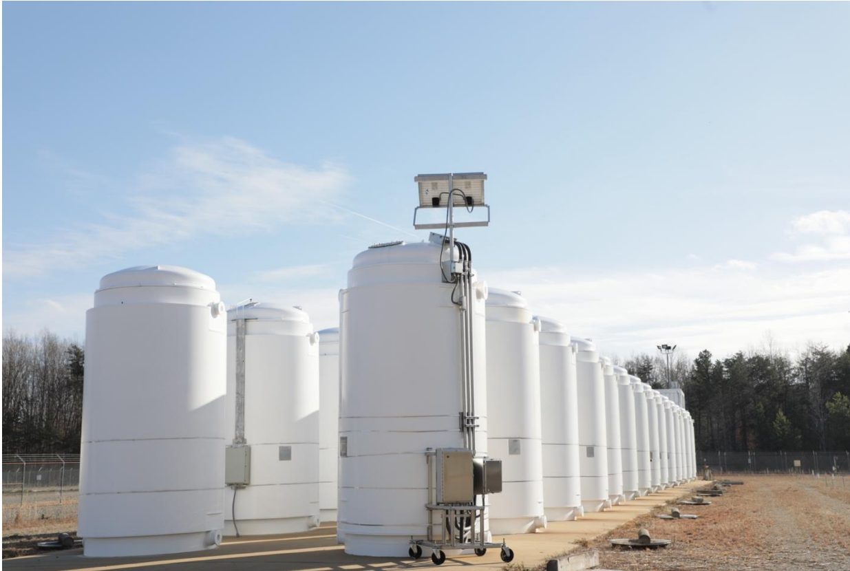
The HBURC shown as currently stored at the North Anna Power Station. The temperature measuring equipment that distinguishes it from the other casks will be removed prior to shipment to Idaho National Laboratory.
