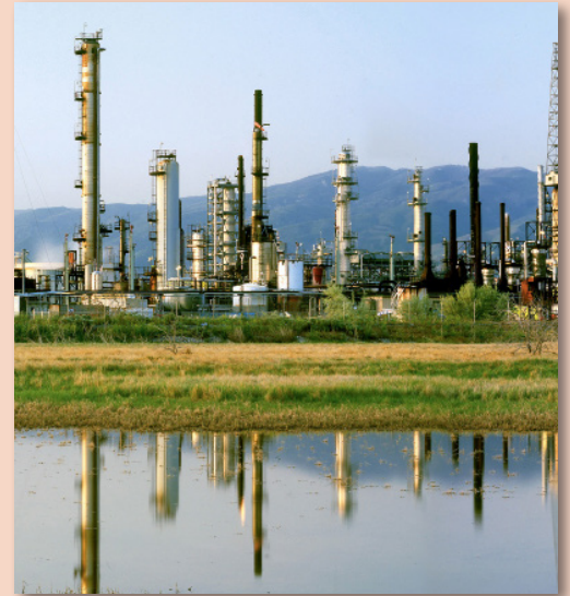
Chevron Refinery, Salt Lake City, Utah
