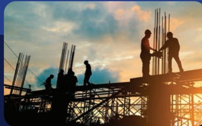
▲ Construction team working
