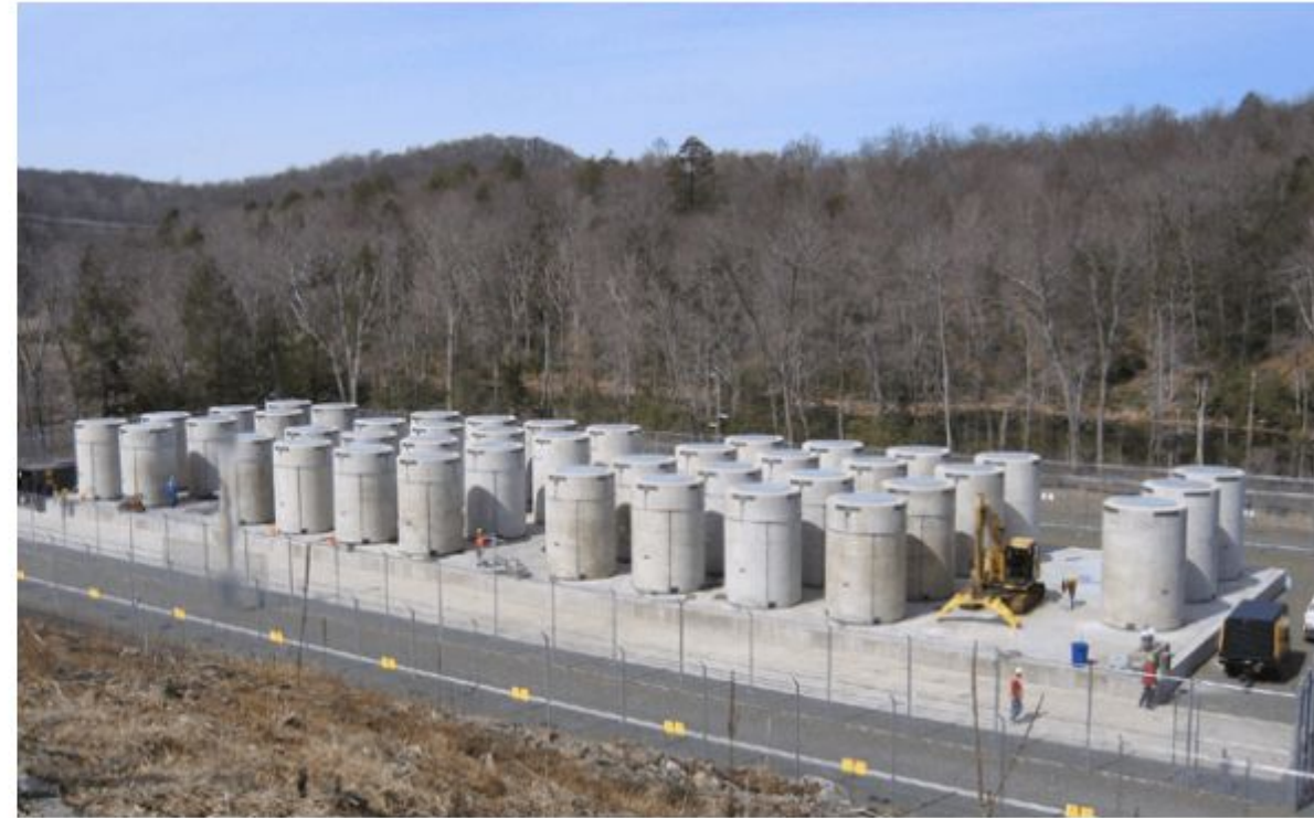
Dry Cask Storage Used at Connecticut Yankee
